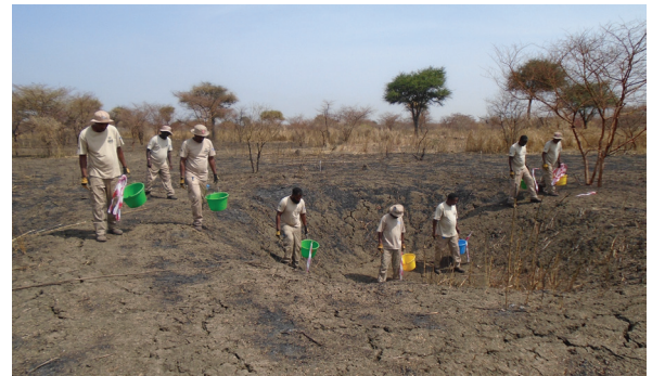
Remediation of the former temporary demolition site in Nyanchour
