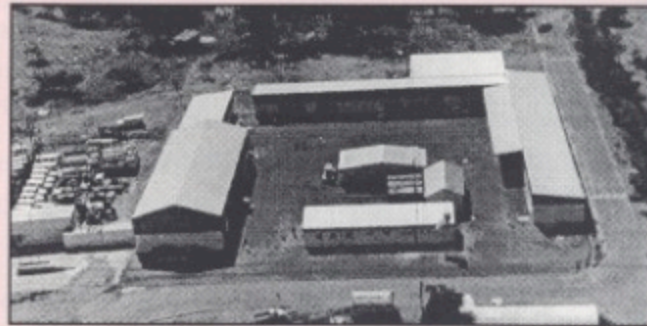
An aerial view of the new complex
